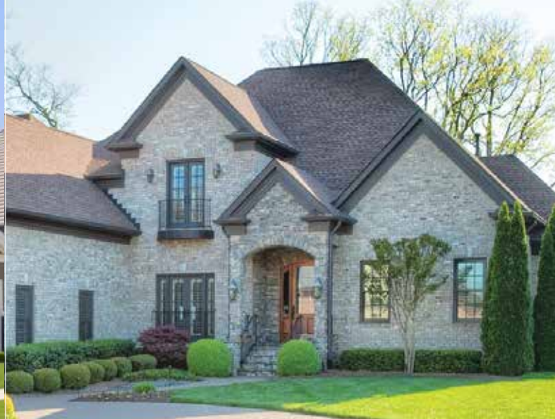
Sliding Door Replacement
