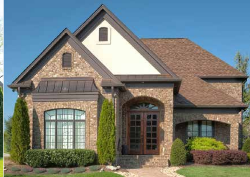
Swing Door Replacement
